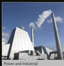
Power and Industrial
