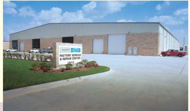
▲ The new 20,000 sq. ft. Roots service centre in Houston, Texas.
